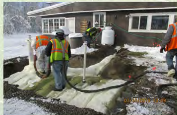
Construction crew installs a belowground water storage tank for potable water.
